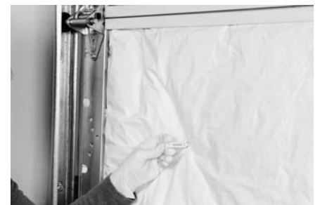
Install Retention Clips
