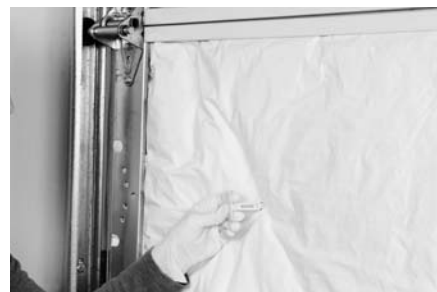
Install Retention Clips
