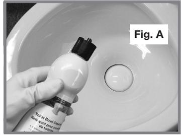
**FLUSH BALL CLEANING:** After a period of time, mineral deposits from hard water may build up on the flush ball or seal, resulting in a slow water leak. To prevent this, periodically clean the flush ball and seal.
