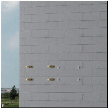
④ Cut holes in the wall against the chassis of the pole.
