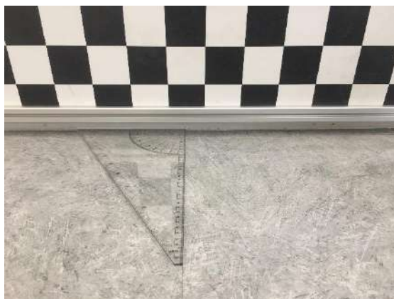
Finding a line perpendicular to the wall
