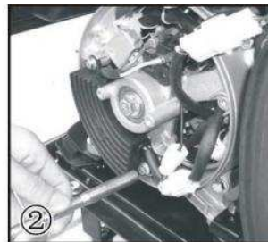
② Remove the 2 bolts (M5x16) holding the AVR.
