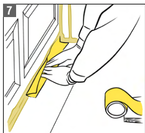
7 Seal door to foundation with Tape, pushing fold into seam.
