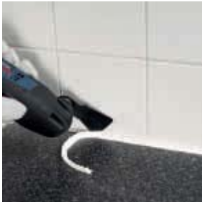
Removing old silicone joints.
