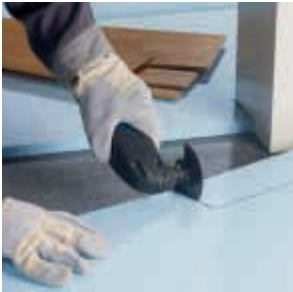
Cutting tread sound insulation plates to size cleanly and efficiently.
