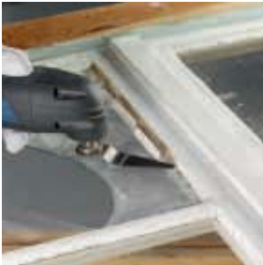
Cutting window putty (sealing compound).
