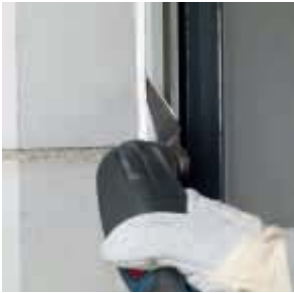
Cutting soft expansion joints.
