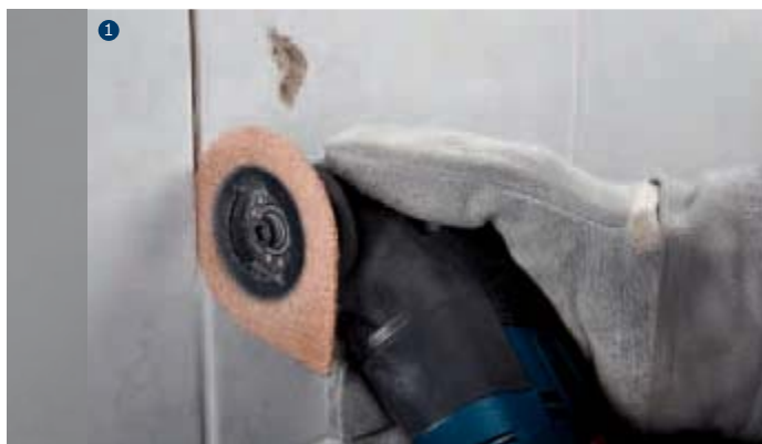
1 Routing joints on wall and floor tiles.
