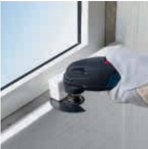
Cutting protruding insulation material, e.g. polystyrene, flush.
