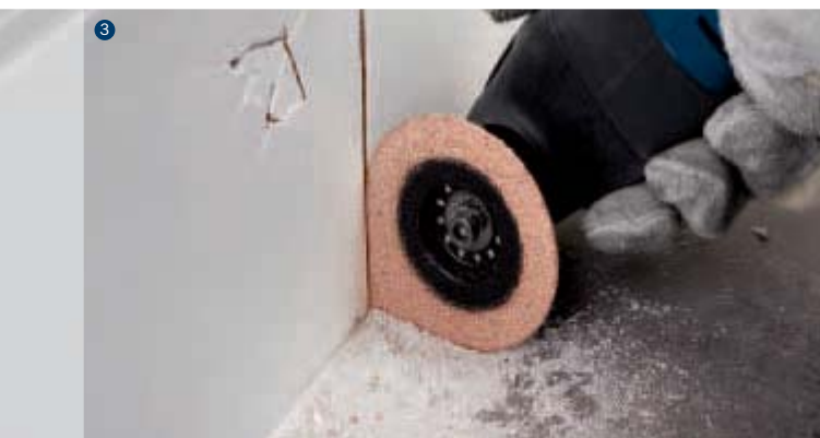
Routing joints right into 90 degree corners.
