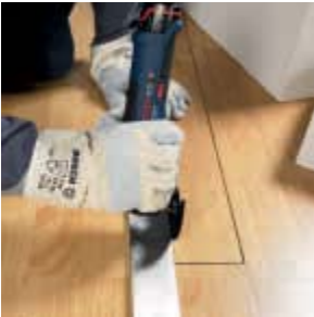
Cutting out laminate/parquet accurately, e.g. for installing a partition wall.
